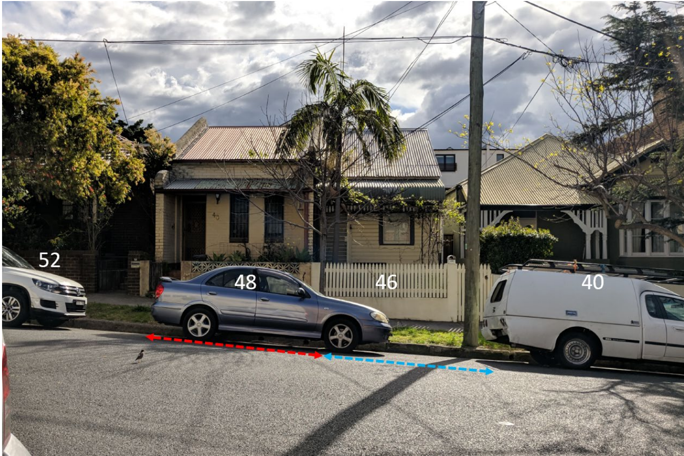
46 Victoria Street and 48 Victoria Street
